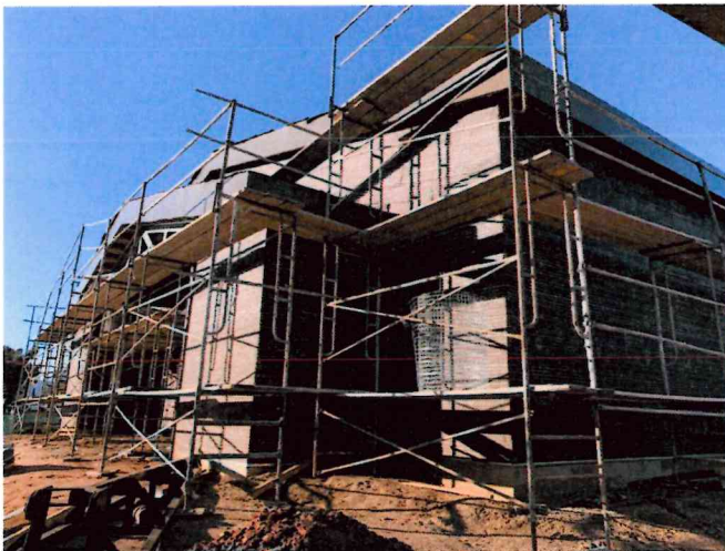
Lindo Park – Multipurpose Room and Kitchen Modernization
