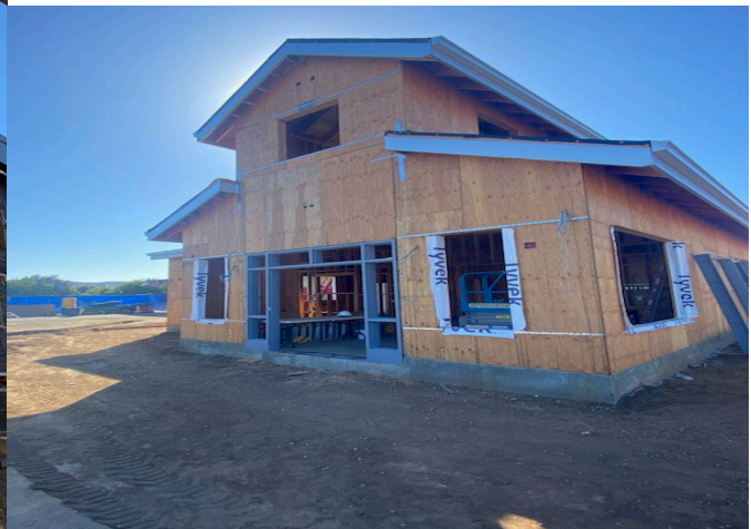
Lakeside Farms – Administration Office, Bathroom, and Kitchen Modernization
