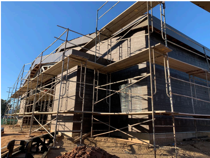
Lindo Park – Multipurpose Room and Kitchen Modernization
