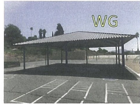
Eucalyptus Hills Winter Gardens Shade Structure
